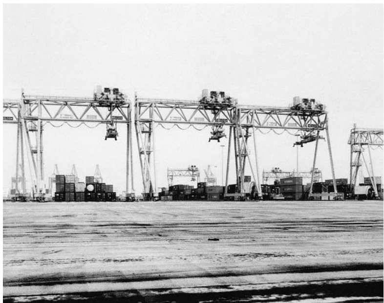
Fig. 6.13.1 ASCs with Spreader Positioning Systems
