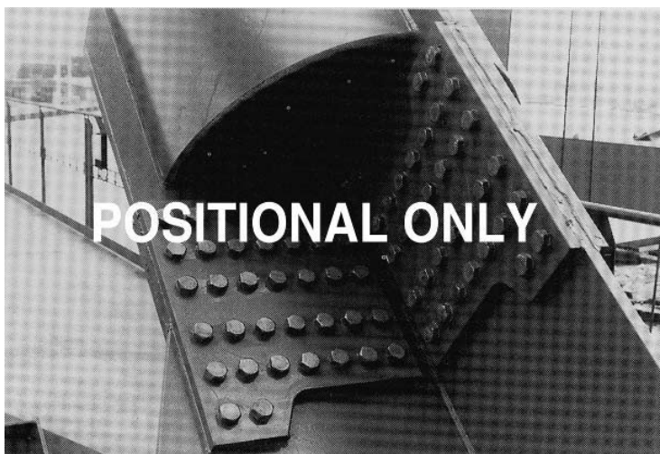
Fig. 7.5.8 Bolts in a back tie
