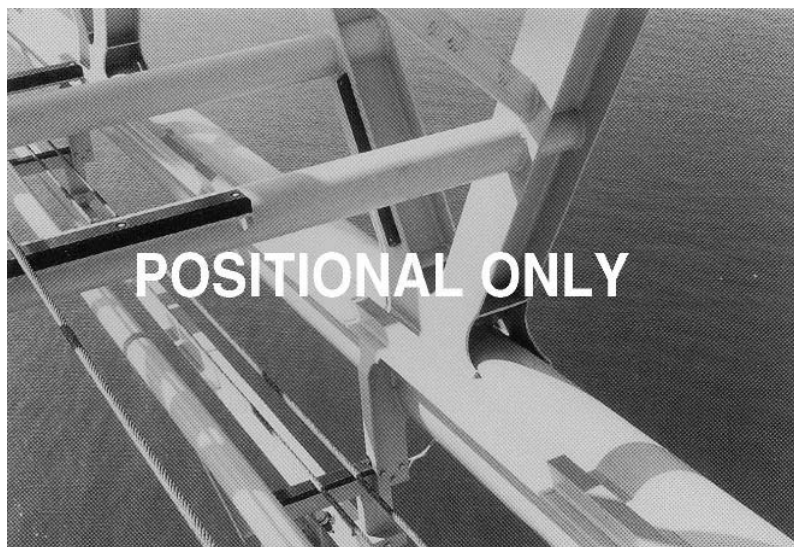
Fig. 6.1.3 Fully supported wire ropes
