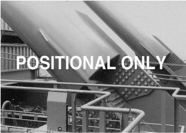
Fig. 7.3.1 Bolted connection
