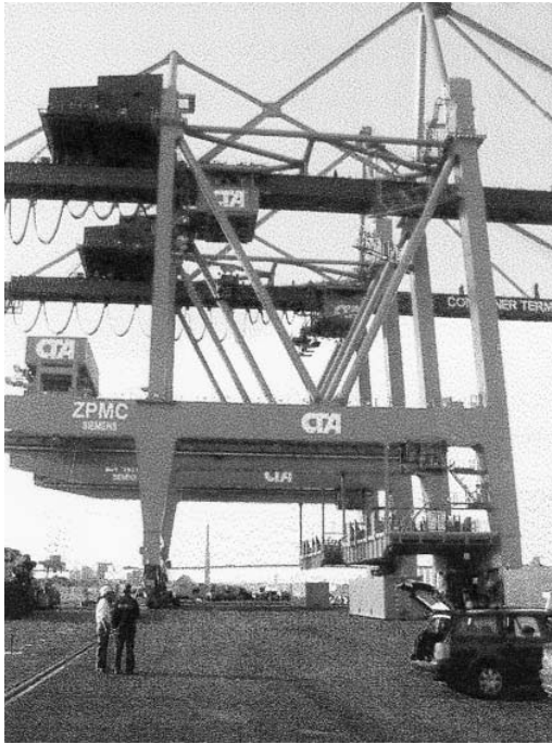
Fig. 6.12.3 Crane with laser scanners
