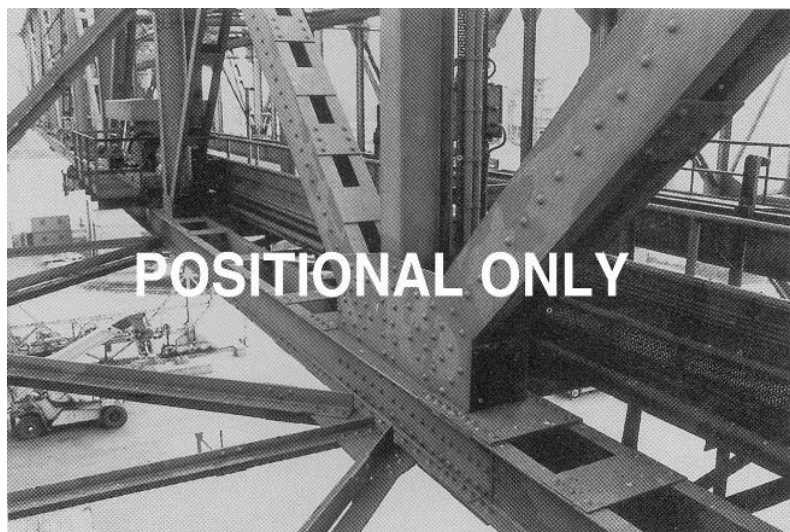
Fig. 7.4.2 Riveted construction
