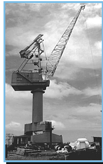
Fig. 8.5.14. 10 te capacity shipyard wharf crane
